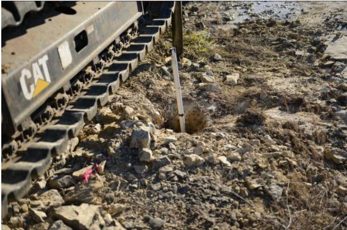
Figure 6: Piezometer installation.
